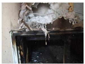
Figure 5 – The burn pattern at the air return duct.
