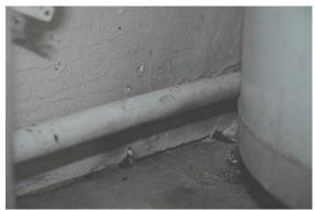
Figure 9 – The 3/8-inch gap above the floor board of the water heater and furnace closet where the natural gas entered the closet on the day of the fire.
