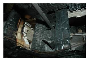
Figure 6 – The area where the gas line entered the end of the insulation-filled wall cavity.
