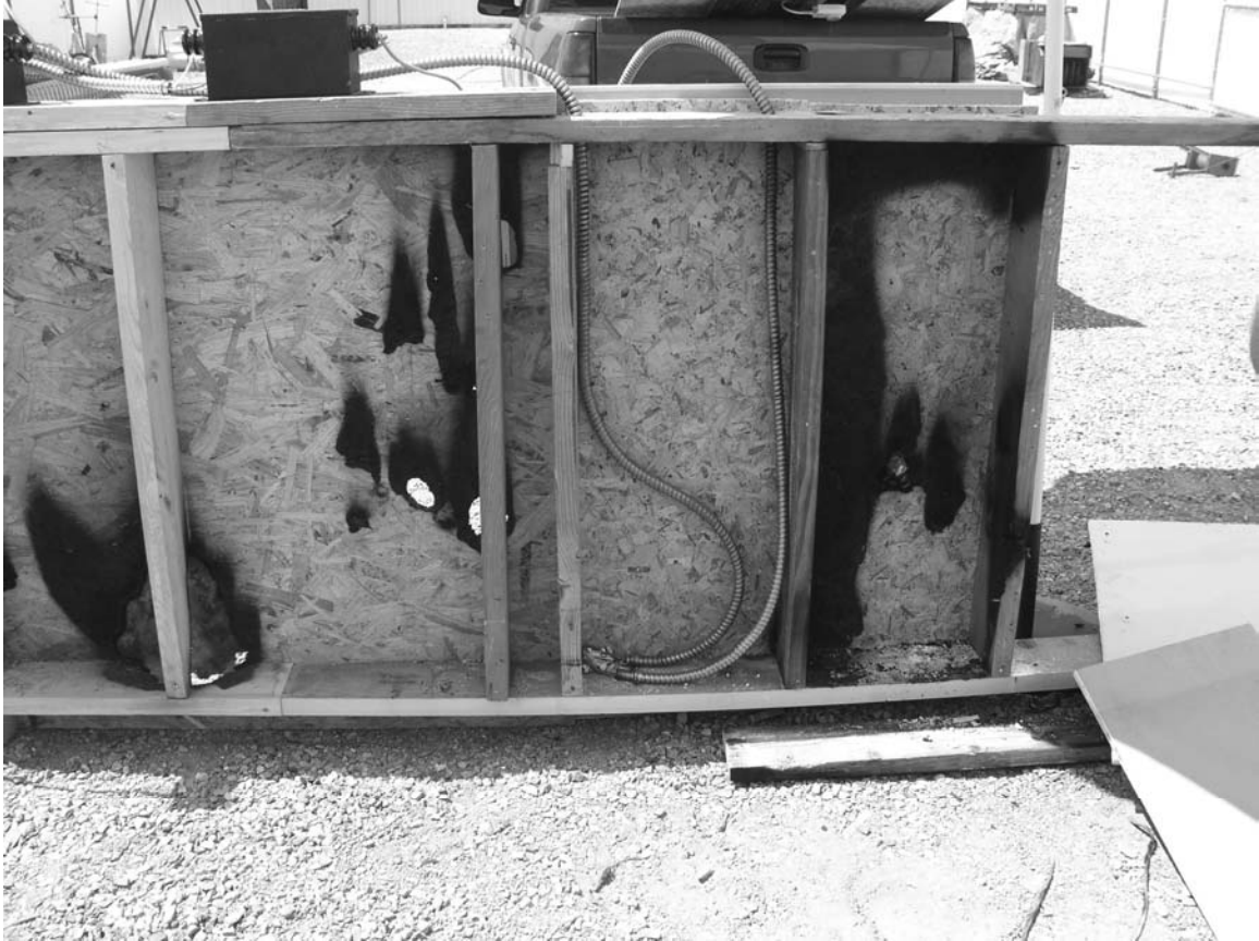
Figure 8 - Neon transformer testing burn patterns
